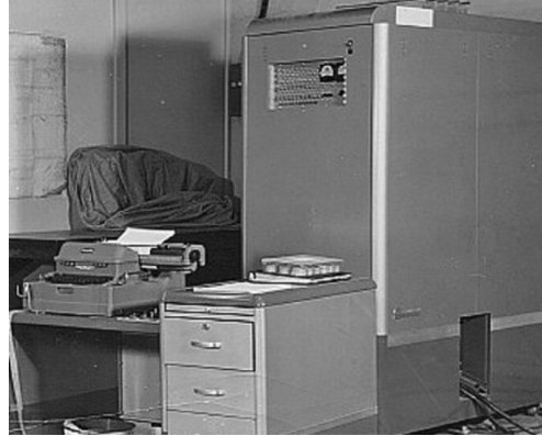
Figure 1. The NCR 102-A system installation at the Royal Canadian Air Force Station (now called Canadian Forces Base) in Cold Lake, Alberta.
